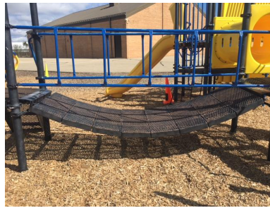
Bridge is breaking/ platform is bent
